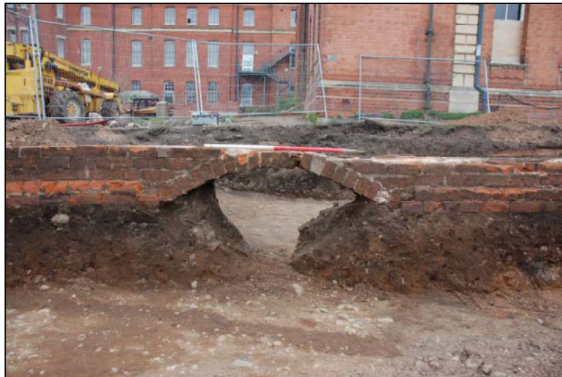
Figure 19: Relieving arch in late post-medieval garden(?) wall (2023). Scale at 1m, facing north.
